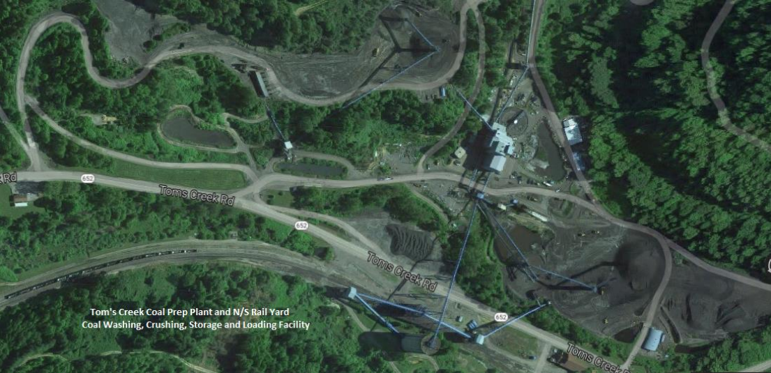
Figure 1: Tom's Creek Coal Prep (cleaning) and Railroad Loading Facility
